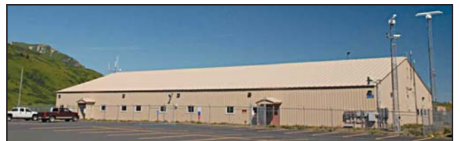
The Launch Control Center
