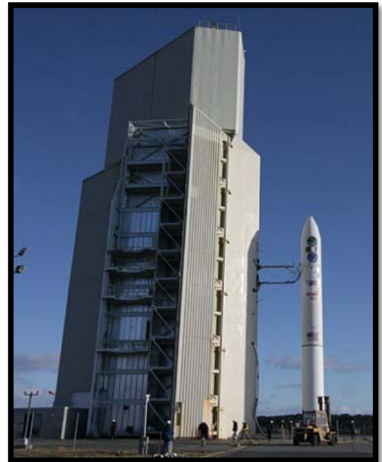
KLC Launch Pad 1
